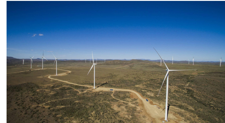
Noupoort wind farm in Northern Cape has 35 wind turbines
